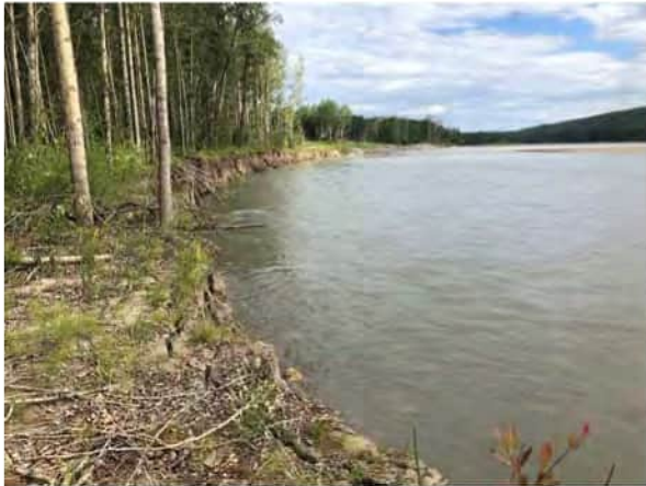
a) View looking upstream at eroding bank between bridge and pipeline right-of-way.
