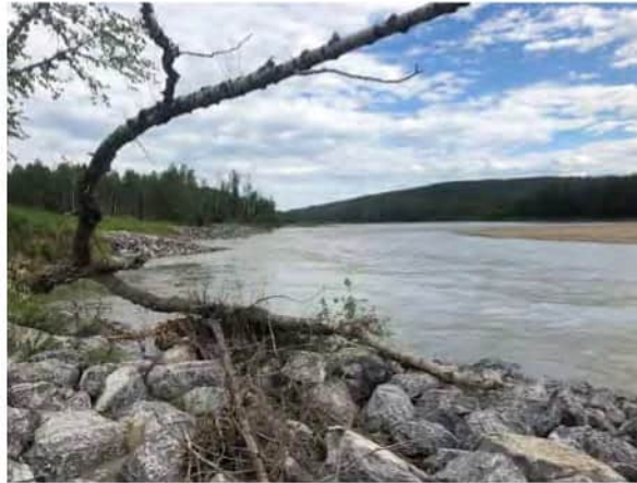
b) View looking upstream at rock spurs at pipeline right-of-way.
